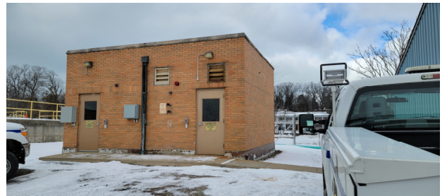
Chemical Feed Building to be Demolished
