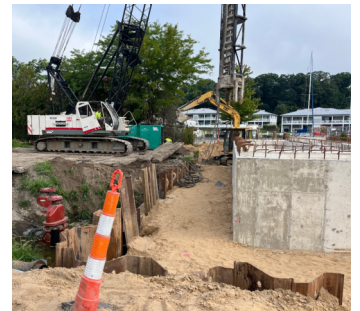
UV Structure Auger Cast Piles
