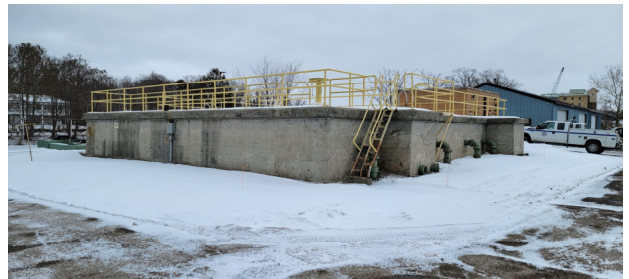
Chlorine Contact Tank to be Demolished
