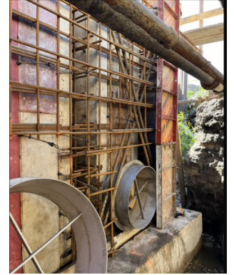
Flow Split Structure Construction
