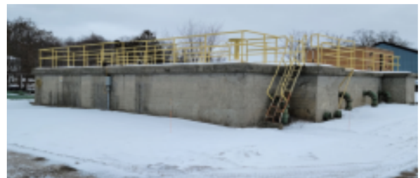
Chlorine Contact Tank to be Demolished
