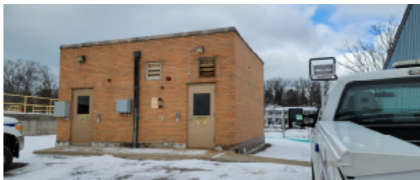
Chemical Feed Building to be Demolished
